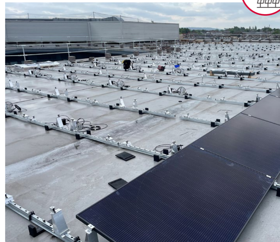
Solar panels being installed on Regent Point
