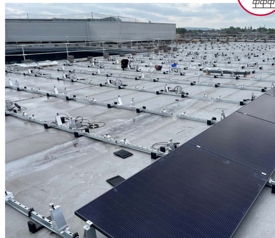
Solar panels being installed on Regent Point
